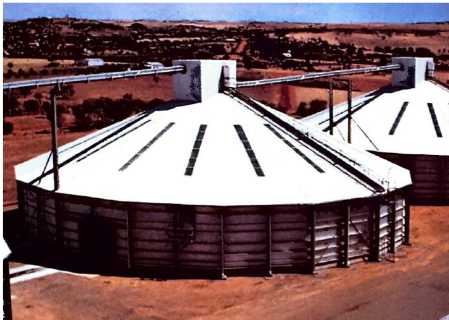
Figure 27: The “M Type” grain silos Northampton, 1990
