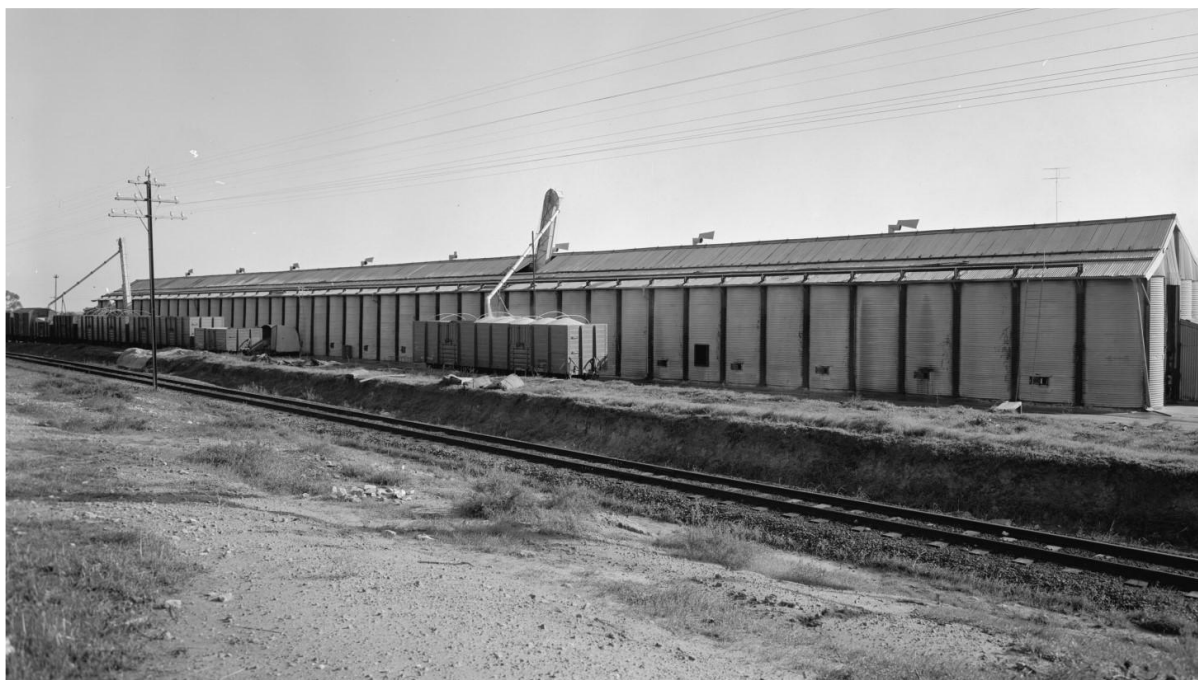
Figure 15: Wheat Rail Loading Silo at Cunderdin, 1963
